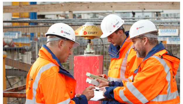
Establishment of a primary grid using high-precision GNSS measurements
