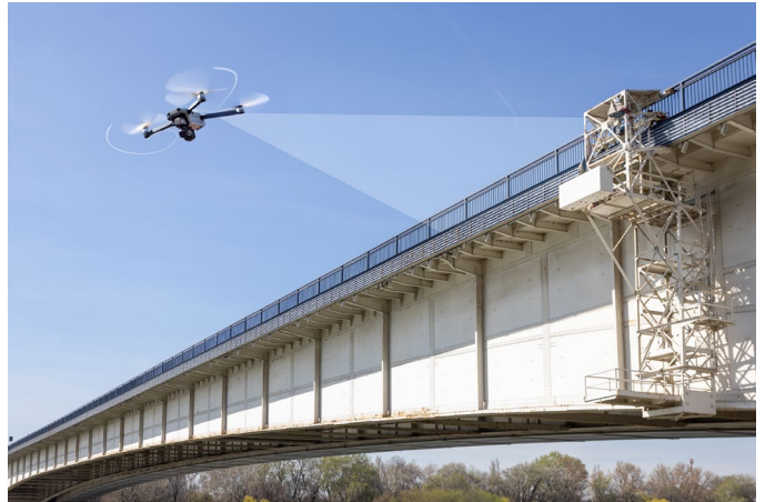
UAV surveying: as-built documentation and inspection of bridges
